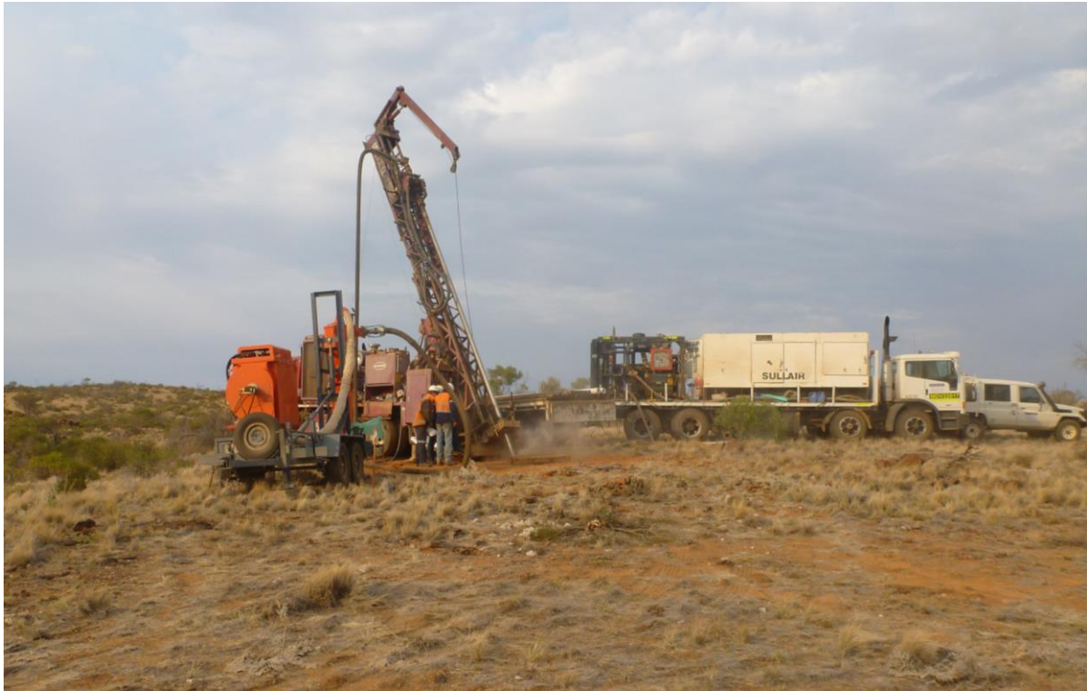
Figure 1. Core Exploration's RC drilling on the Scott Lee Prospect, Fitton Project, South Australia.
